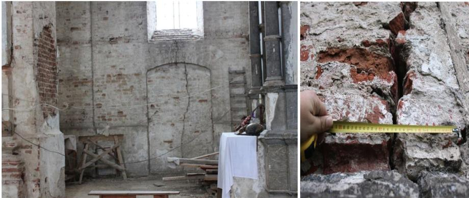
Fig. 6. A view of the damage of the interior wall from inside the building (photograph to the left) as well as a close-up of a visible crack in the structure of the wall (photograph to the right).
