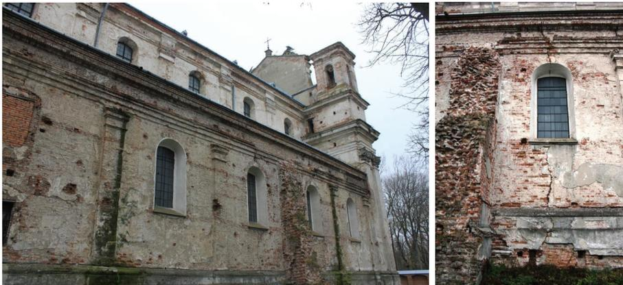
Fig. 7. The photograph depicts the building from the eastern side (photograph to the left). Visible damage of the abutment of the wall, along with the material and structural degradation of the wall (photograph to the right).
