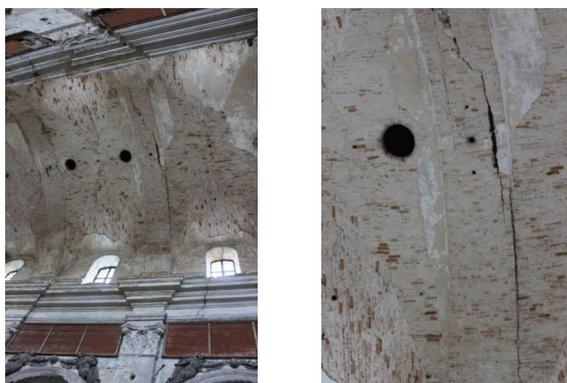
Fig. 5. A view of the cracks and marks on the vault ceiling (photograph to the left), as well as a close-up of the damage (photograph to the right)
