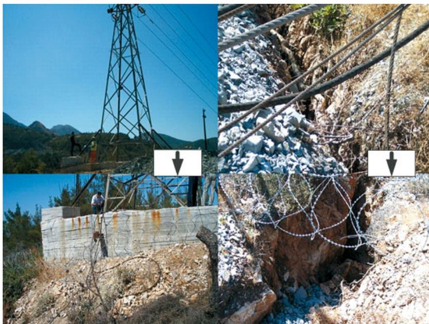
Fig. 7. Preview of subsidence effects on Pylons (No: 18-19)
