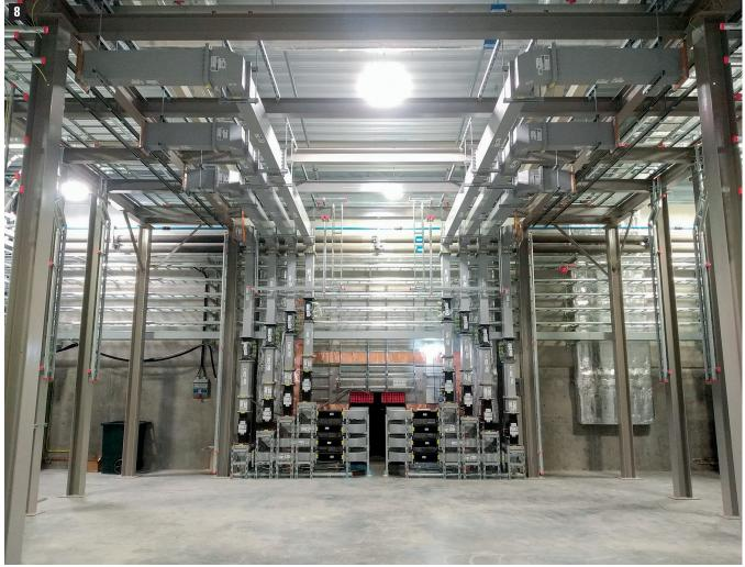
Fig. 8 Power distribution system – waveguides 704 MHz ready for tuning
