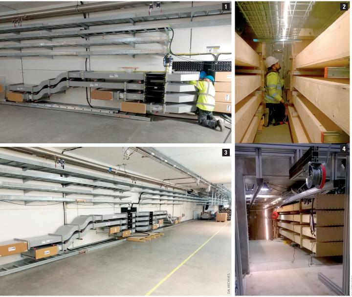
Fig. 1 Waveguide installation in the accelerator tunnel
