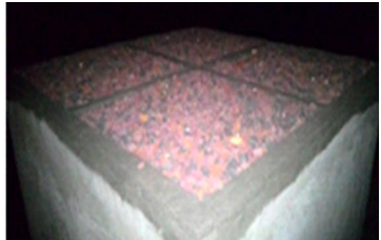
Fig. 7. Roof slab with Jhama brick bats.
