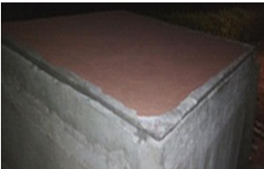
Fig. 5. Rubber sheet roof slab.
