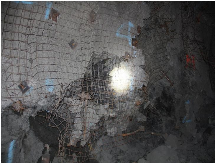
Fig. 6. A rockburst case at diamond mine
