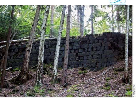
A wall made of cast slag blocks.
