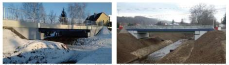
Fig. 8. First Polish vehicle bridges made of FRP materials in service: all-composite (left) and hybrid (right).
