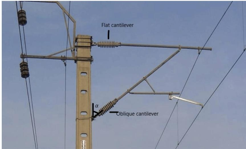
Fig. 1. Installation layout of cantilever insulator
