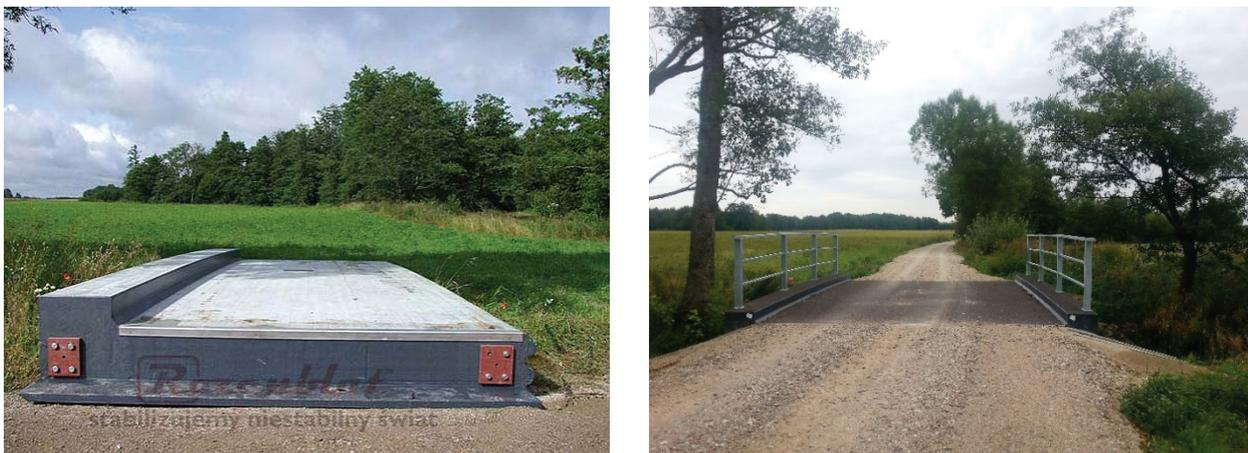
Fig. 8. Bicycle bridge of the Dutch InfraCore system in the commune of Lelkowo: half of the slab structure; finished object [12]
