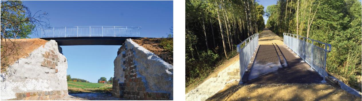
Fig. 9. Bicycle footbridge of the Dutch InfraCore system in the commune of Kiwity [12]
