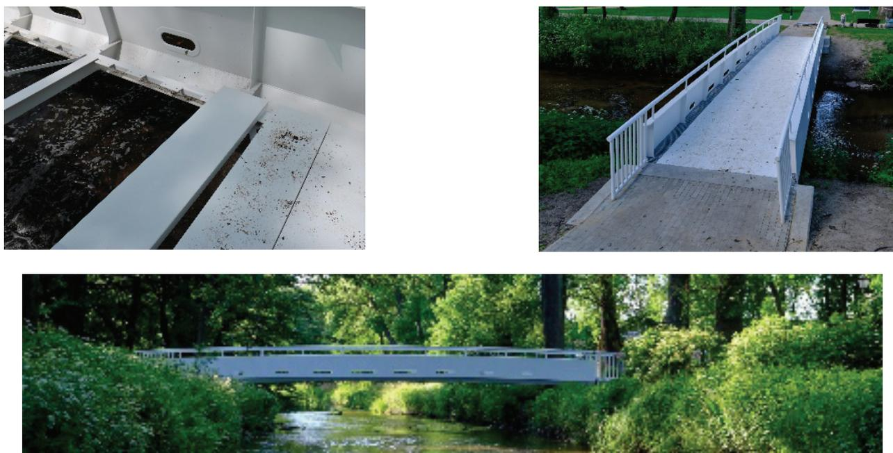
Fig. 16. FRP panels, top view and side view of the footbridge [8]
