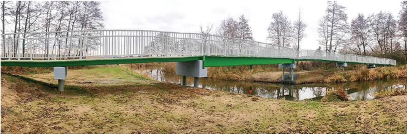
Fig. 11. Bicycle footbridge of the Dutch InfraCore system in the commune of Frombork [12]
