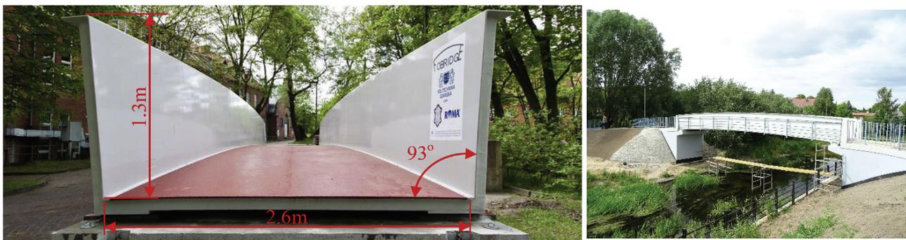
Fig. 7. Footbridge in Pruszcz Gdański: a) cross-section of the span; b) general view on site [1, 2]
