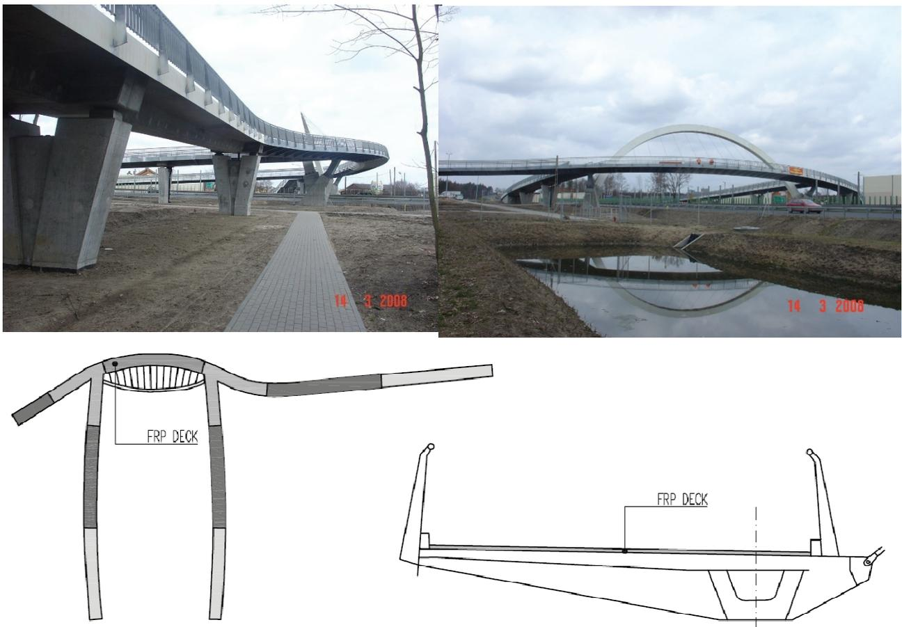
Fig. 14. View and cross section of the main span with FRP deck [6]
