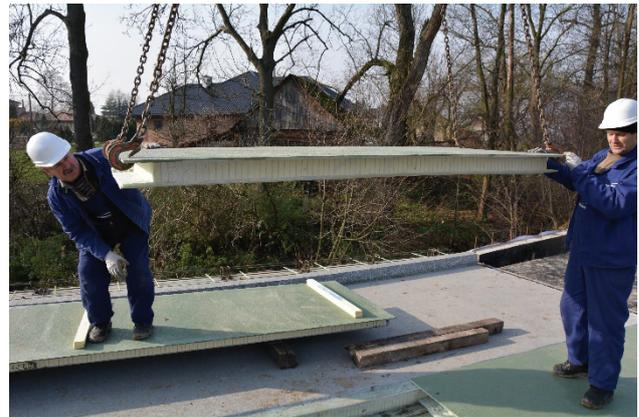
Fig. 17. Footbridge under construction and cross section of the main span with FRP deck
