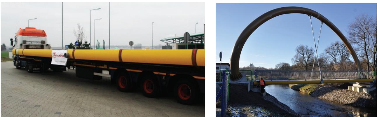
Fig. 10. Bicycle footbridge of the Dutch InfraCore system in the commune of Gołdap – transport of the span and general view [12]
