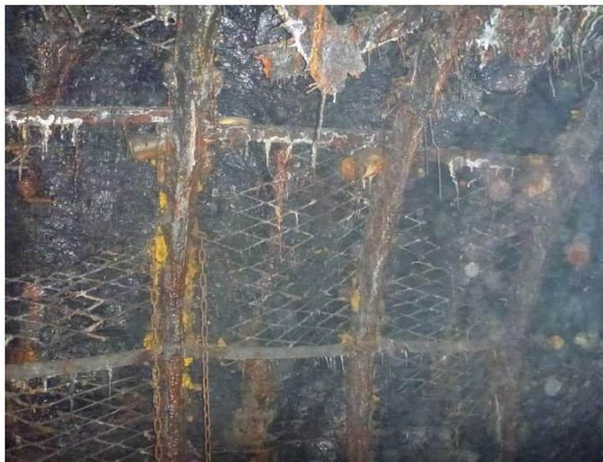
Fig. 2. Corroded MM mesh lining
