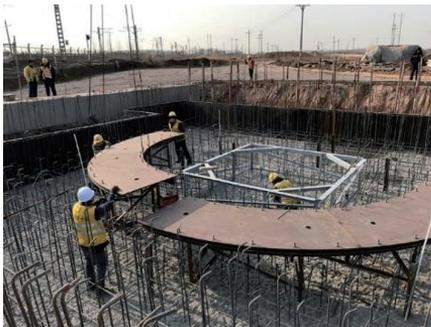
(c) Spherical hinge and ring road construction
