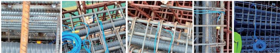
(a) Embedded sensors in various parts of the bridge
