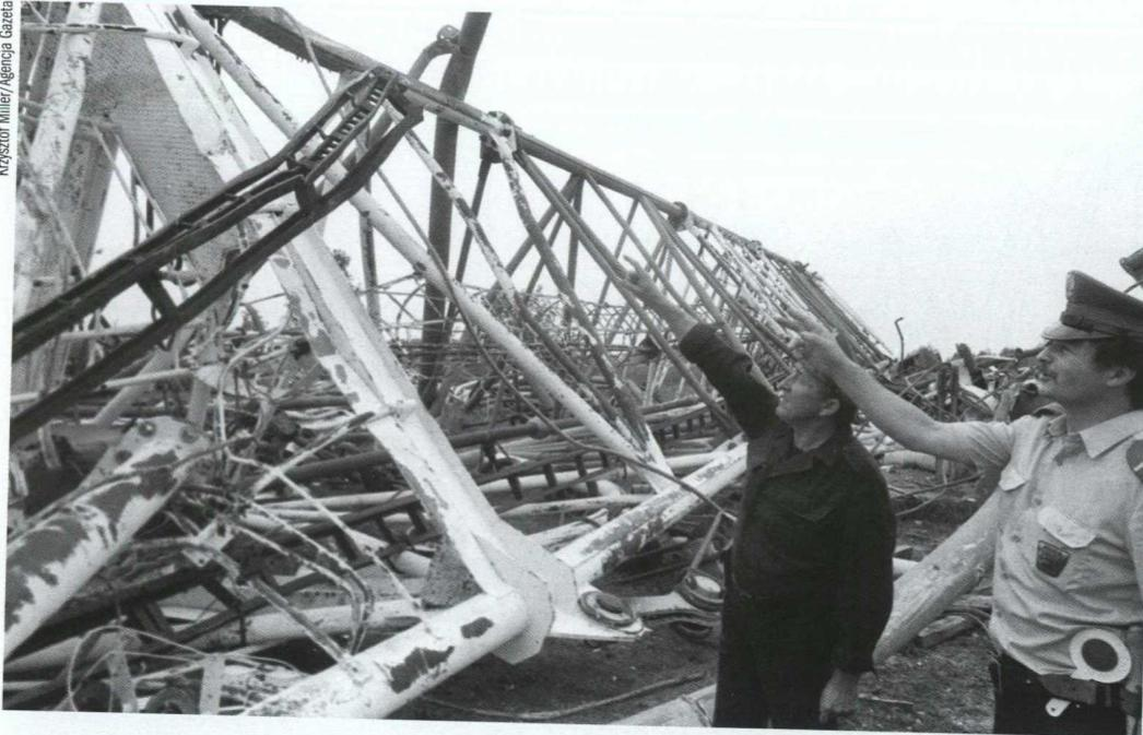
646.38 meters tall, the antenna came online in 1974. Conservation work that was begun in 1991 disturbed the statics of the antenna core, which collapsed on 8 August 1991. The job of broadcasting Polish Radio 1 was taken over by two antennas in Solec Kujawski near Bydgoszcz, only 330 and 289 meters tall
