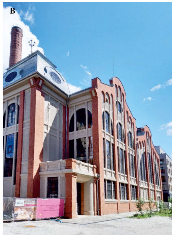
Ill. 9. Karol Scheibler's Art Nouveau power plant from 1910, built to a design by Alfred Firsch. The oldest building within the borders of the then Kingdom of Poland in reinforced concrete frame construction. A) State of preservation (2017). B) As seen after the revitalization (2023) Photos by A.A. Tomczak.
