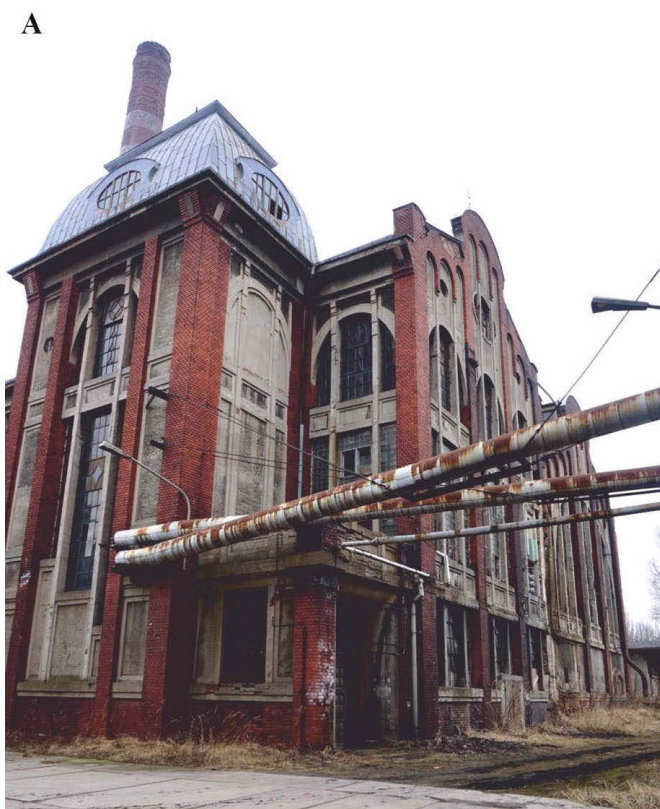
Ill. 9. Karol Scheibler's Art Nouveau power plant from 1910, built to a design by Alfred Firsch. The oldest building within the borders of the then Kingdom of Poland in reinforced concrete frame construction. A) State of preservation (2017). B) As seen after the revitalization (2023) Photos by A.A. Tomczak.
