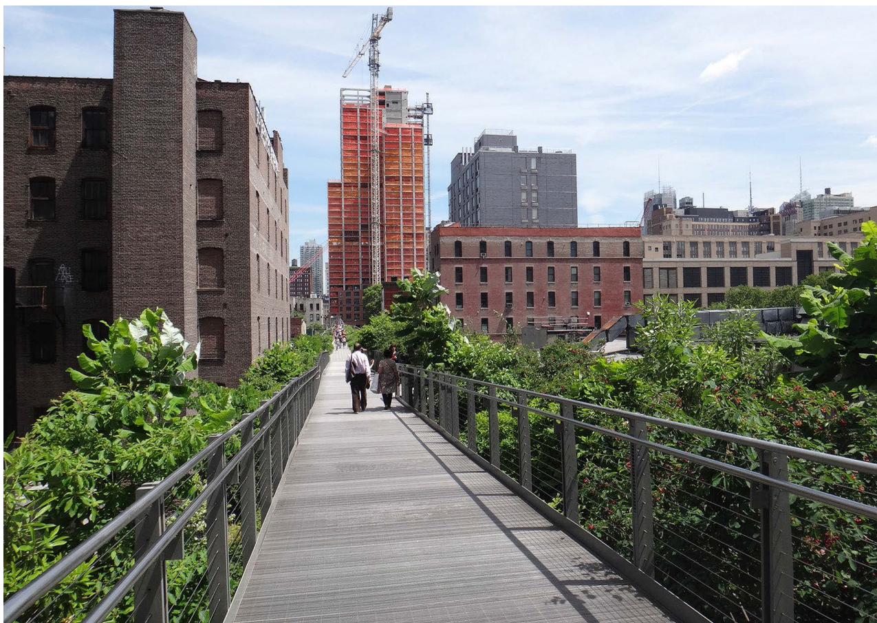
Ill. 3. View of the pedestrian bridge in High Line Park — a walk among the treetops below the overpass. Photo by A. Pięt.
