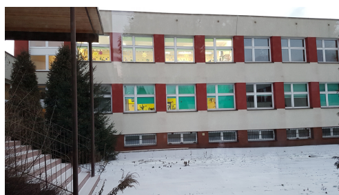
Fig. 1. East elevation of analysed school building
