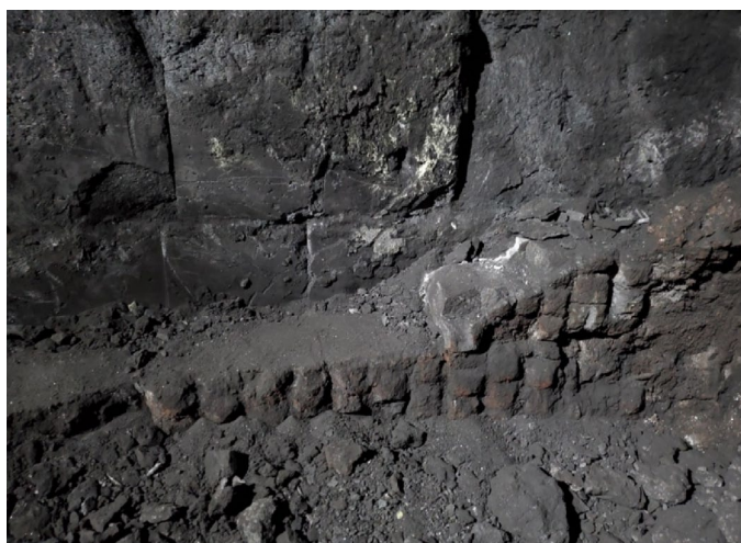
Fig. 5. Photo of Saint-Gobain ceramic tumbler residue at the level of the 8th row of carbon blocks of BF-8 at «Arcelor Mittal Kryvyi Rih»
