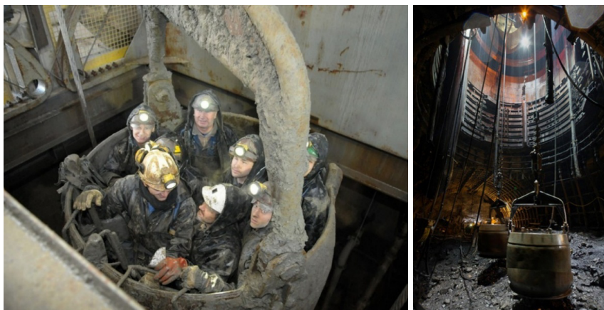
Fig. 3. Transport in a shaft under construction (hoisting system) [8,9]
