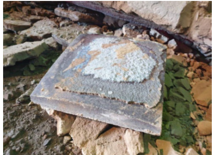
Fig. 8. Top view of the impact pad after casting, with no visible deformation and surface coating present
