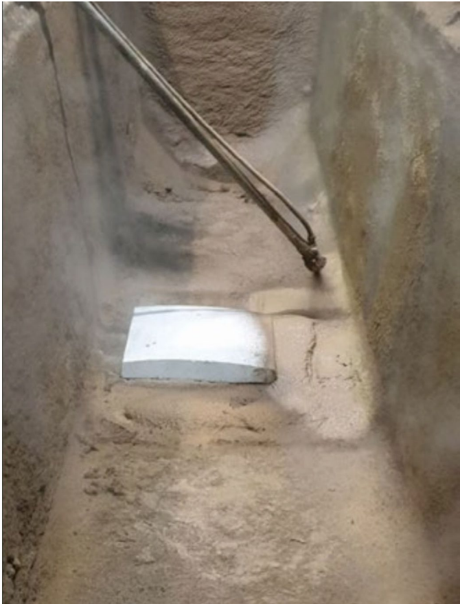
Fig. 6 Installing the prototype spherical impact pad in the tundish before casting
