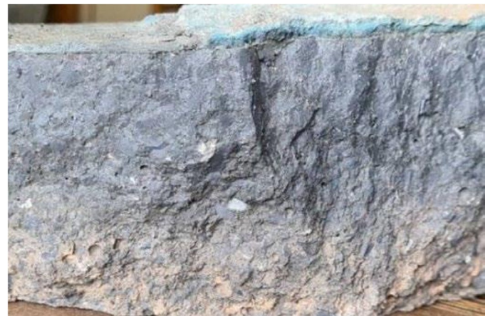
Fig. 9. Surface Condition at the Point of Steel Impact on the Impact Pad
