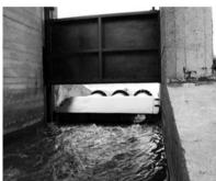
Fig. 2. Hypolimnion discharge channel with the Olszewski tubes
